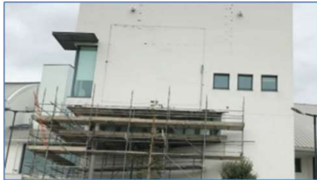
(d.) View of Scaffolding erected @ Cube 25.02.20 & Banner Removed
